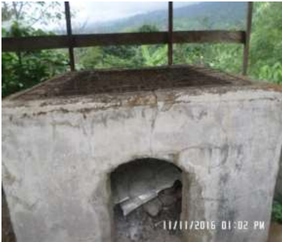
A fish dryer. It consists of concrete walls and a fire place. The top has strong metal rods on which the fish is placed.
