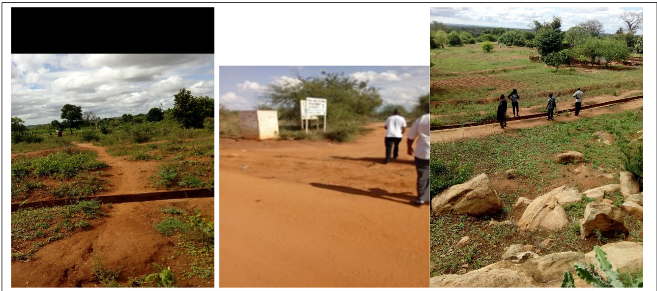
Abandoned Drip Irrigation Infrastructure at Masimbani and Kake
